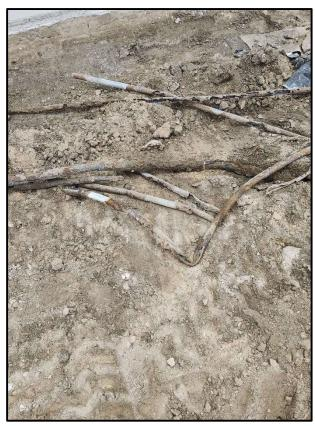
Rusted/Broken Conduit Under Concrete
