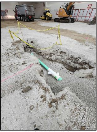
New Drain Tile Installed
