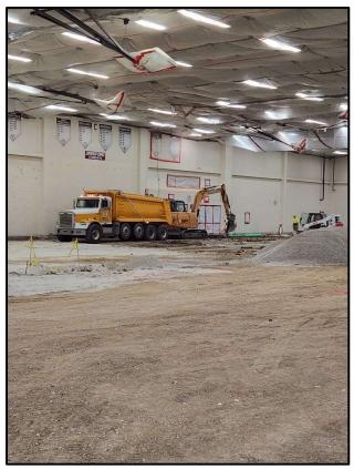
Interior Excavation for New Drain Tile
