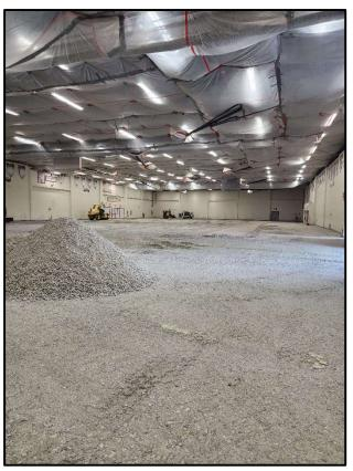
Backfilled & Graded for New Concrete Subfloor
