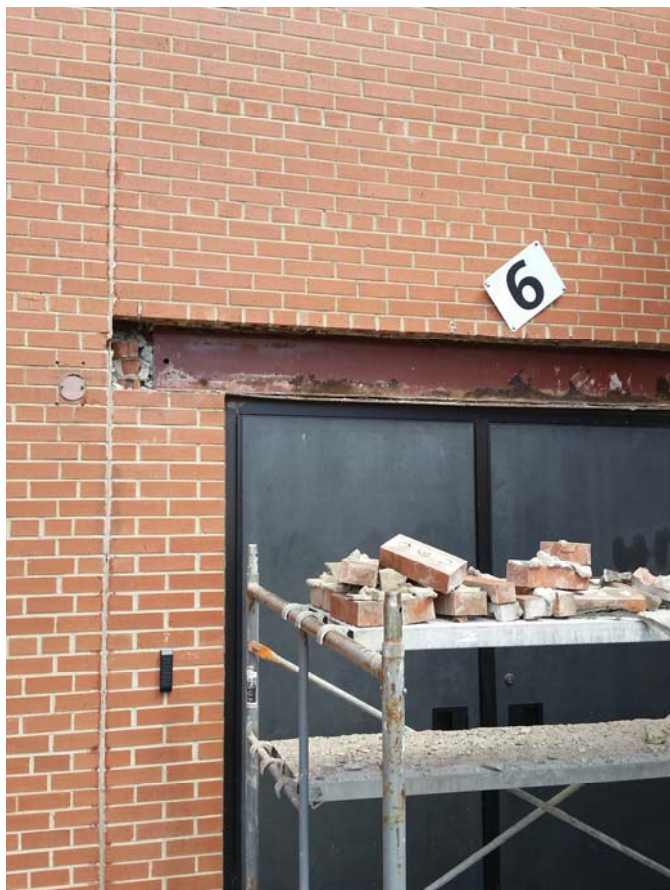
ALICE Door Replacement at Jefferson and Tremper masonry repairs
